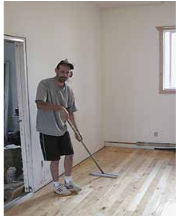
Jens Kugelstadt applying last coat of urethane
