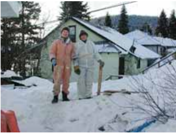
Judy Campbell and Jody Hunter scraping, bleaching and stacking salvaged flooring.
