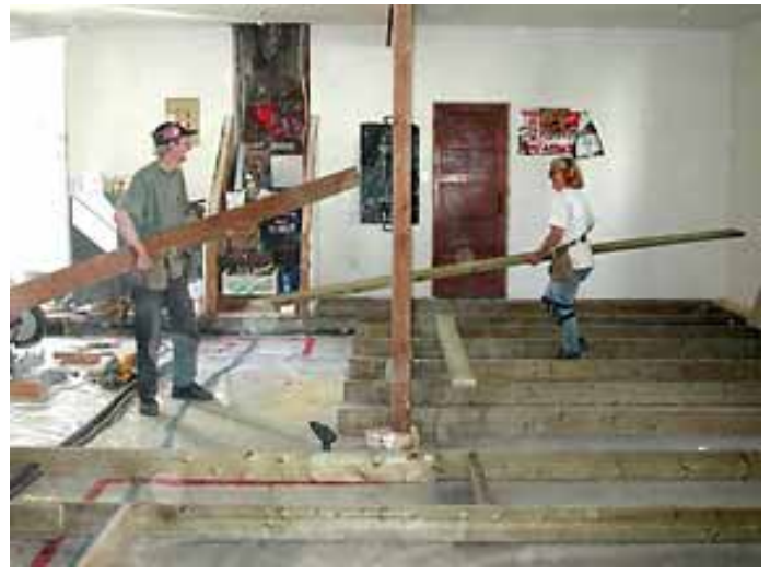
Bill & Maureen Trotter restringing print shop subfloor
