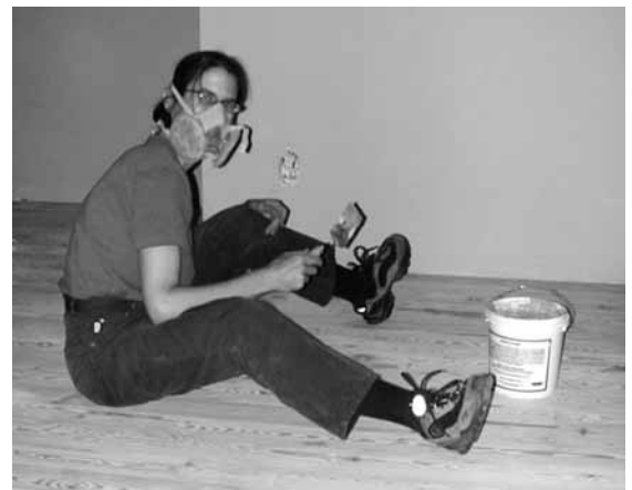
Pippa filling holes in flooring.
