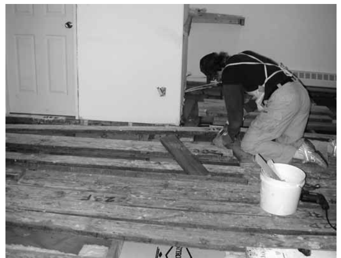
Charlie Roots replanking print shop subfloor
