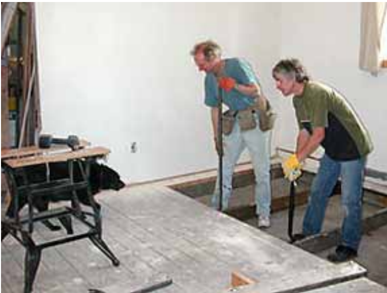
Bill & Sandy Bunce pulling up old den subfloor
