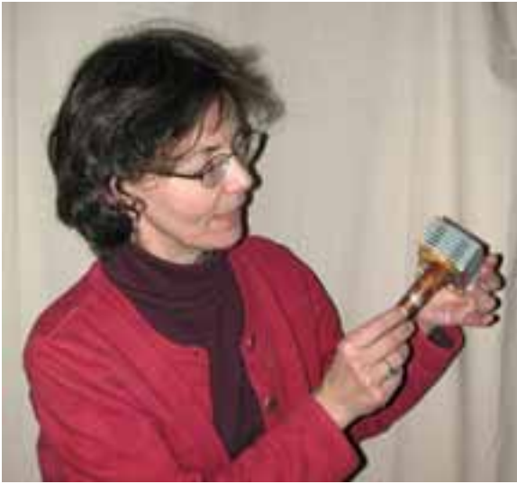
Claire with a piece of burst copper baseboard line.
