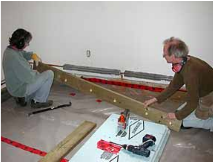
Bill & Sandy Bunce nailing new plate to concrete.
