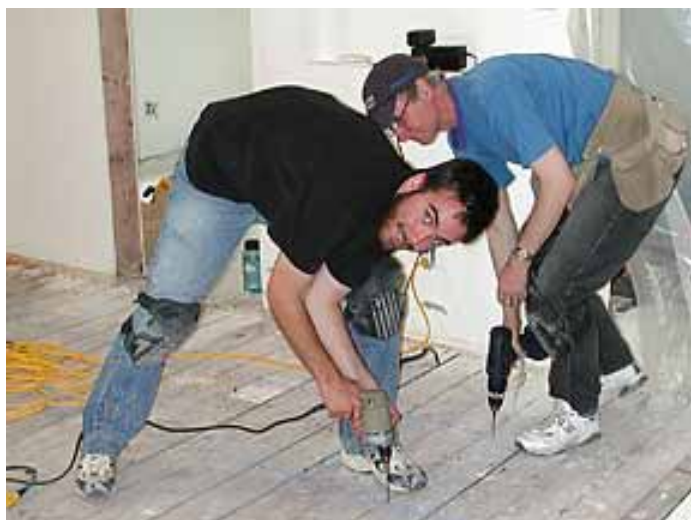
Steve Ross & Bill screwing around with the decking
