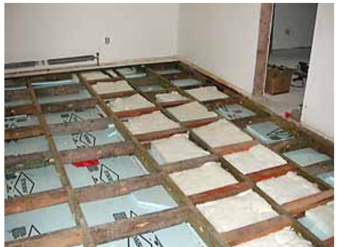
repaired, insulated print shop subfloor
